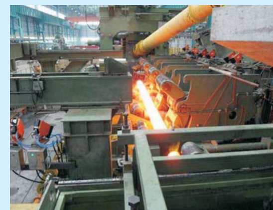
Seamless pipe hot-rolling mill Capacity: 300,000 MT/year
